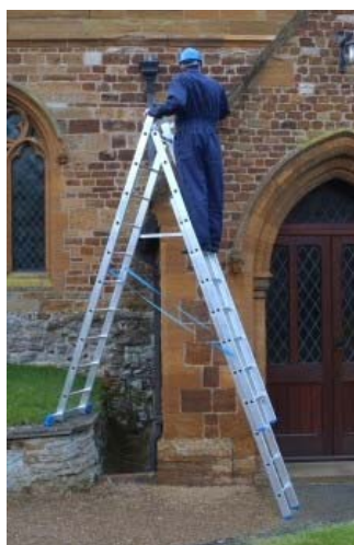
It's a stairwell ladder ...
