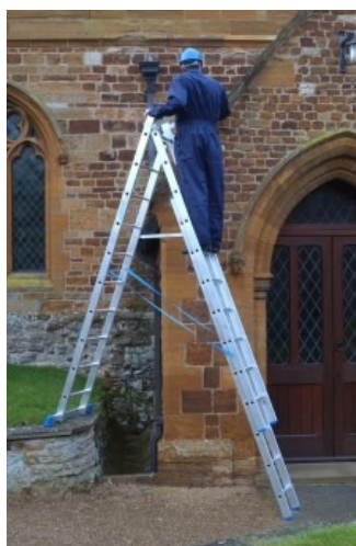
It's a stairwell ladder ...
