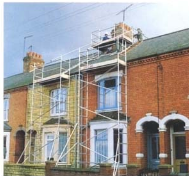
Walk-Through base frames for pedestrian access under tower.
