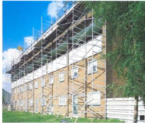
Bridge Beams between single and double width towers.
