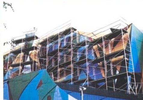
Special scaffold of single width towers.
