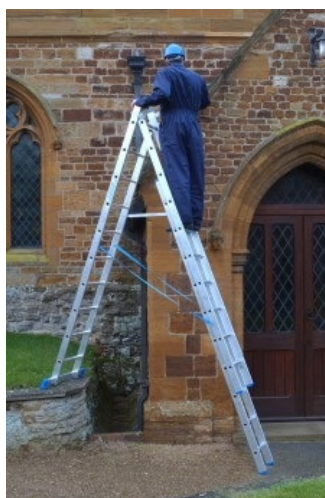
It's a stairwell ladder ...
