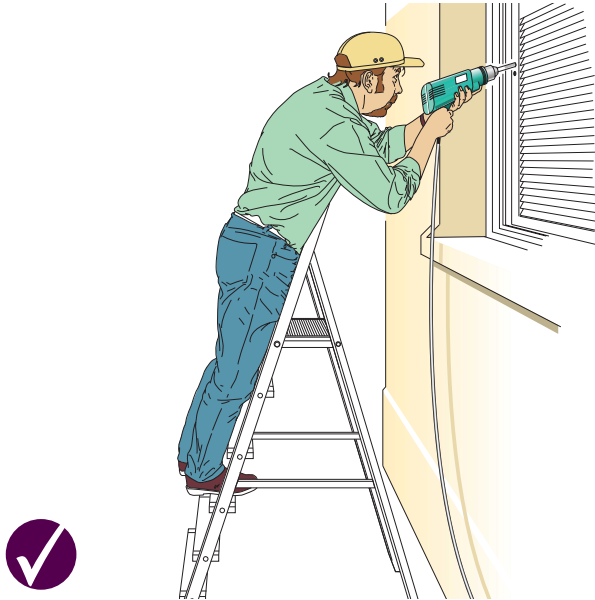
Figure 3a Correct - rungs facing work activity
