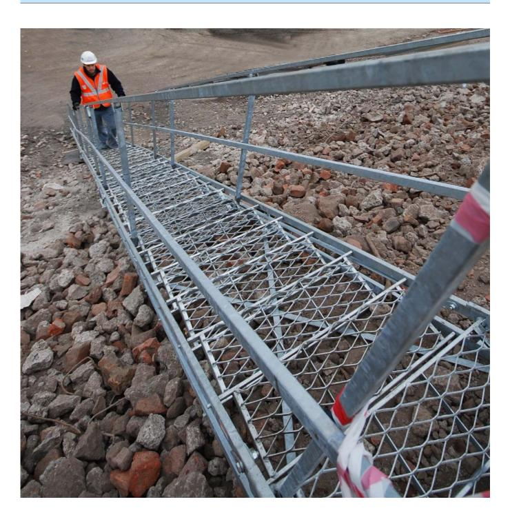
Fast & secure temporary embankment stairs.
