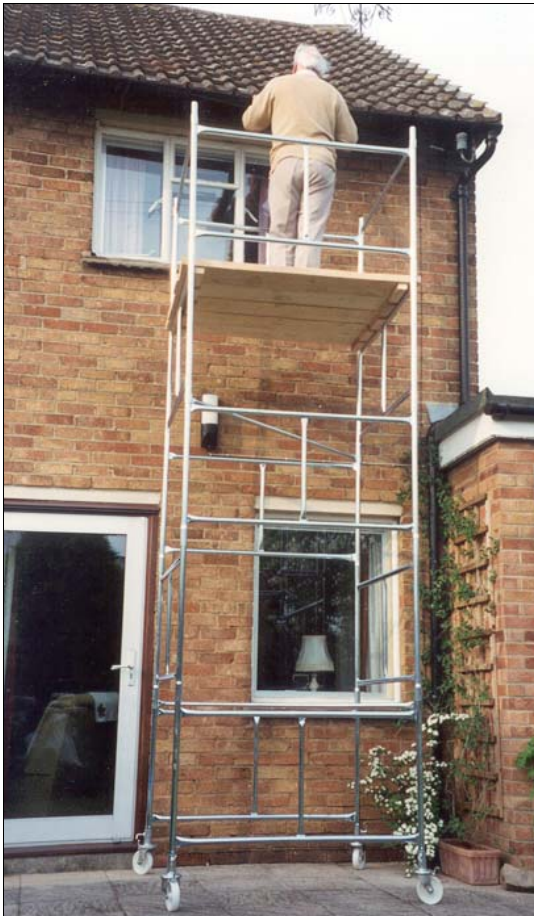
Domestic Tower 4' x 4' base size. Safe & easy. Shown above is a 10ft platform height tower which gives comfortable reach to a standard 16ft gutter.
