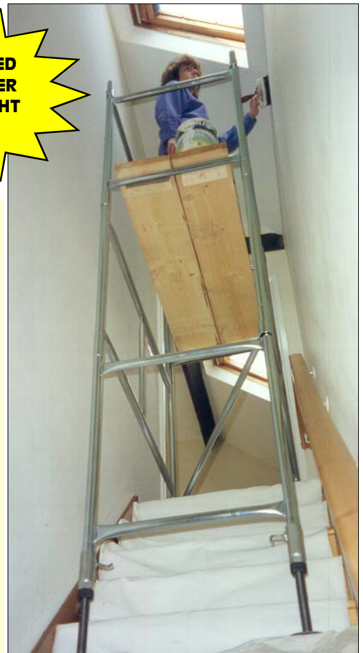
Domestic Towers can be converted into scaffolds to provide safe access in most stairwells. Much safer than flimsy steps and scaffold boards!
