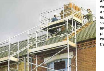
Although few customers bother with it, we would point out that to comply with Health & Safety regulations, some form of scaffold (e.g. alloy towers or tubular steel scaffolding) should be erected at eaves level to provide the extra safety of edge protection for employees as they are carrying Klikstak components up & down the roof ladders
