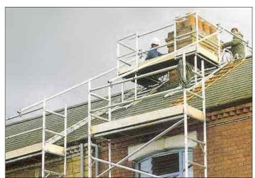
Although few customers bother with it, we would point out that to comply with Health & Safety regulations, some form of scaffold (e.g. alloy towers or tubular steel scaffolding) should be erected at eaves level to provide the extra safety of edge protection for employees as they are carrying Klikstak components up & down the roof ladders
