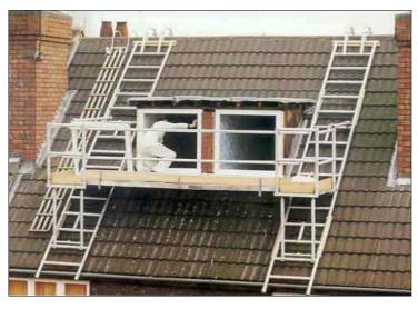
Klikstak's excellent versatility means it can be adapted to reach chimney stacks and dormer windows located down the pitch of the roof.
