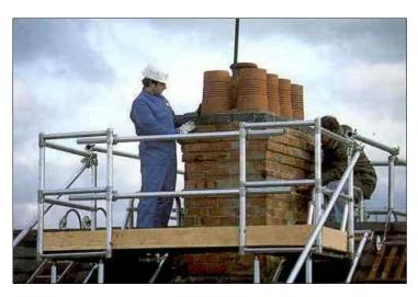
Klikstak is an advanced Chimney Scaffold which is lightweight and easy to assemble and safe in use.
