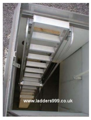
Weight-Assisted ladder here fitted in a 2.3m deep suspended ceiling shaft about 1.1m x 1.1m plan size, giving access to/ from a flat roof.
