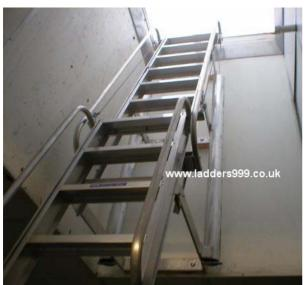
$\,\hat{}\,\,$  ^ counterbalance weights are located inside the alloy tubes at the rear.
