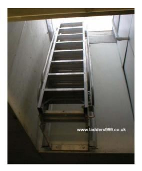
>> the same ladder at the base. Sturdy handrails are fitted to both upper sections.
