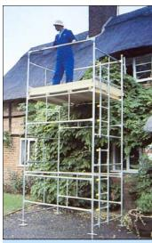
6' x 4' towers give greater platform area and greater reach before having to move the tower, but platform levels can only be fitted at alternate lifts (5'6" intervals) so are not as versatile as the more popular 4' x 4' towers. (Now fitted with double height guardrails - not single height as shown.)
