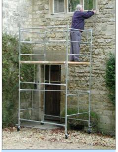
6' x 4' gives greater platform area and greater reach before having to move the tower, but suffers from the disadvantage of platforms only fitting alternate lifts - i.e. standard platform boards will only fit on top of 6ft frames.
