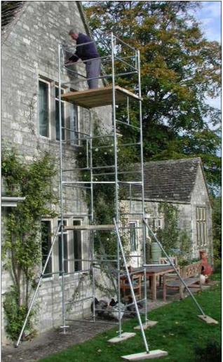
The ever popular 4' x 4' base size shown here with adjustable legs for levelling and a set of stabilizers for extra stability. This platform height of 14' 3" gives reach heights (working heights) up to 20' 3".
