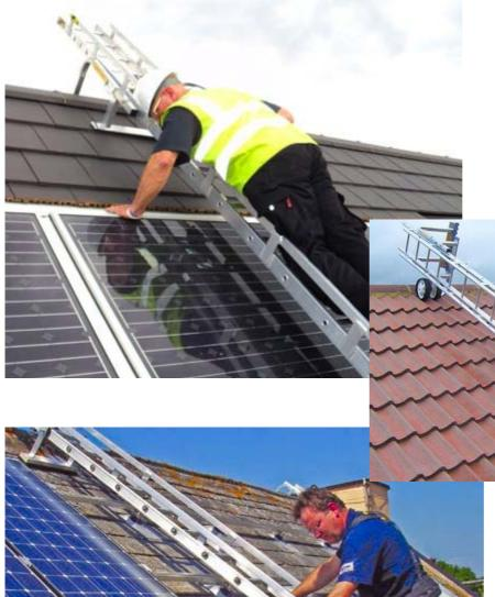
To use, simply roll ladder up the roof on it's soft rubber wheels and then flip 90° into position over the ridge. The special roof hook can be fixed to any rung, enabling the ladder to fit any size roof with the excess length flying the ridge.
