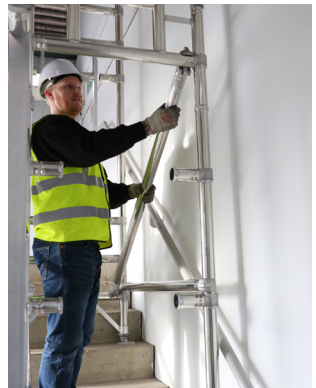
Fit another diagonal from the bottom rung of the plain portal frame to the top rung of ladder portal frame on the right hand side.
