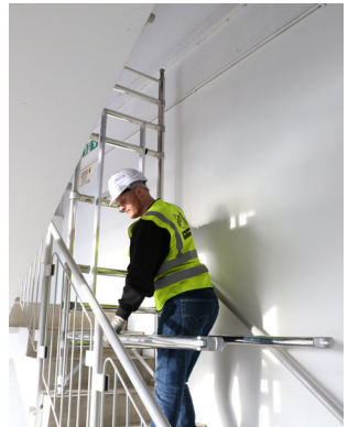
Position the plain portal at the top of your stairs then fit the horizontal braces above the 1st rung.
