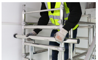
Fit another diagonal from the bottom rung of the plain portal frame to the top rung of ladder portal frame on the right hand side.
