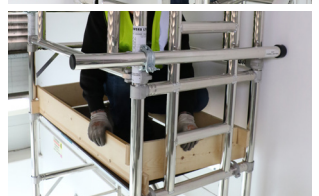
Fit a side prop to the top of each frame, one either end of the tower and then fit your Toe-boards to the tower using the clips.
