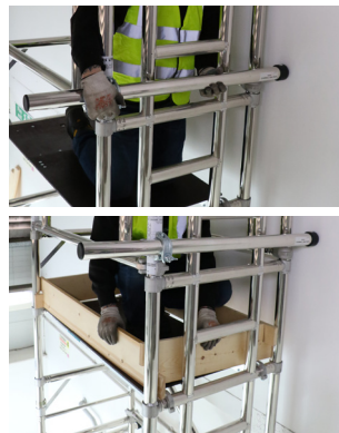
Fit 2 side props every 2m, one either end of the tower. If you cannot fit side props, stabilizers shall be fitted to all 4 corners of the tower. They shall be fitted to create the largest footprint possible. Then fit your toe-boards using the clips.
