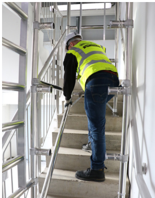
Fit diagonal brace from bottom rung of ladder portal frame to bottom rung of plain portal frame, on the left hand side.
