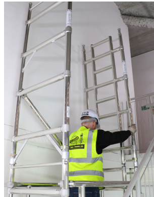
Fit a plain 4 rung frame to the ladder portal frame and engage the interlock clips.
