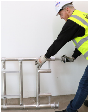
Insert 2 adjustable legs into each of the portal frames
