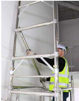
Fit a diagonal brace from the 2nd rung above the platform to the second rung of the 4 rung plain frame.
