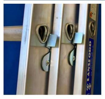
Galvanised rung locks keep sections together when carrying and transporting plus prevent separation when in use but easily rotate for extension. Perfect ladders for most general TRADE activities.
